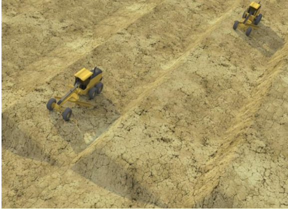
Figure 9: Earthmoving for north-south slopes construction.
